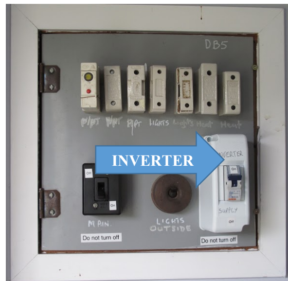
Figure 5: Distribution Board
