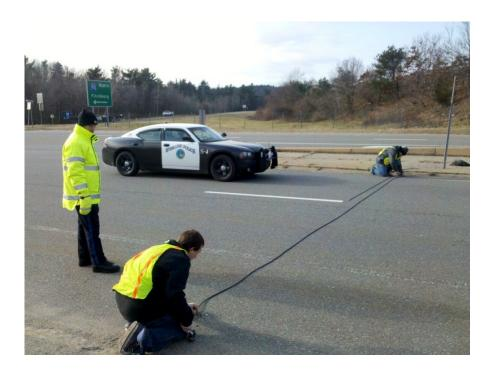
FIGURE 8. INSTALLING ATR TUBES
