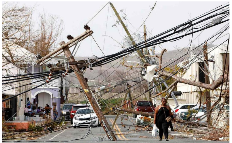
Figure 16. Hurricane Irma destroys power lines (Robin Mejia, 2018).
