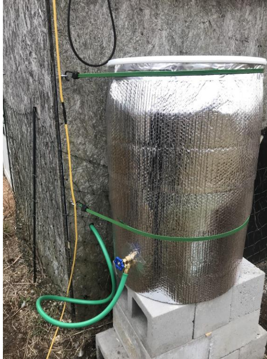
Figure 4. The Barrel outside the Coop. This image shows the set-up of the water storage system outside the coop. The spout, hose connection, insulation, and base of the system are displayed.
