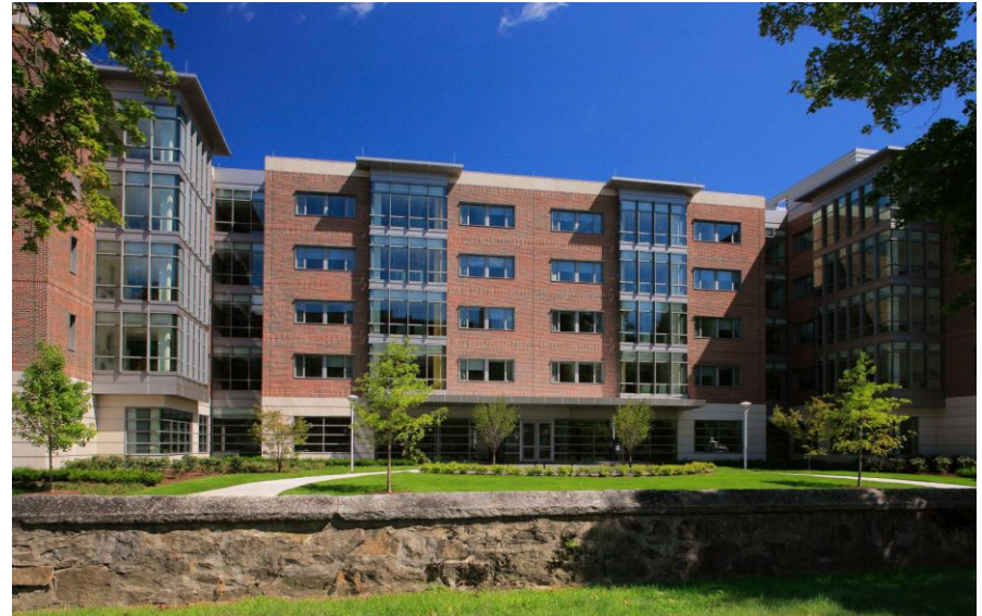
East Hall opened in 2008. It implements numerous sustainability features
