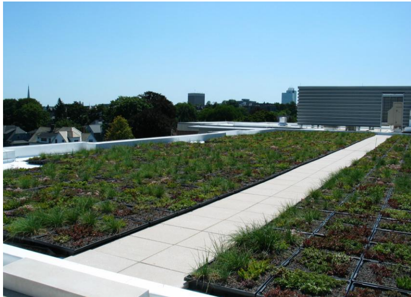
East Hall's Green Roof absorbs sunlight to help cool the building in the summer; it also absorbs water to reduce runoff.
