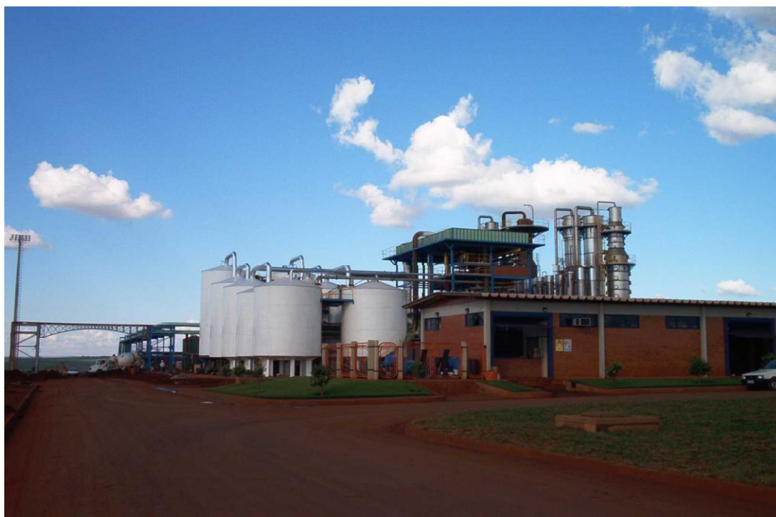
Figure 3.9: Photograph of a group of typical fermentation vats (gray cylinders). The three towers on the far right are distillation towers for the next step in the process (Rediex, 2007).
