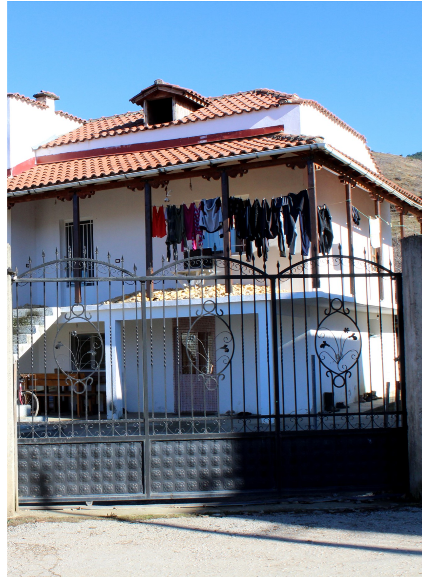
The house of a resident who moved from Old Kamenicë to Lower Kamenicë
