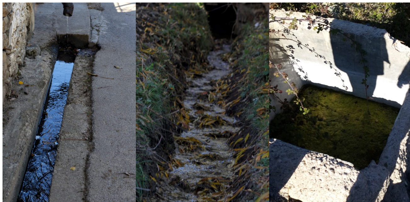
A constructed side channel from Center Kamenicë (Left), Hand dug side channel from Old Kamenice (Center), Picture of a resident constructed septic tank Retrieved Posch & Partners Consulting Engineers et al., (2017) (Right)
