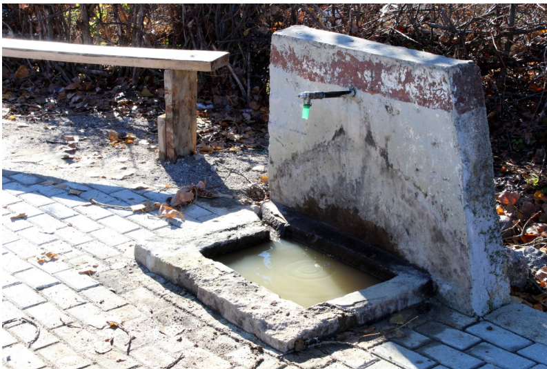
An Outdoor Sink in Kamenicë
