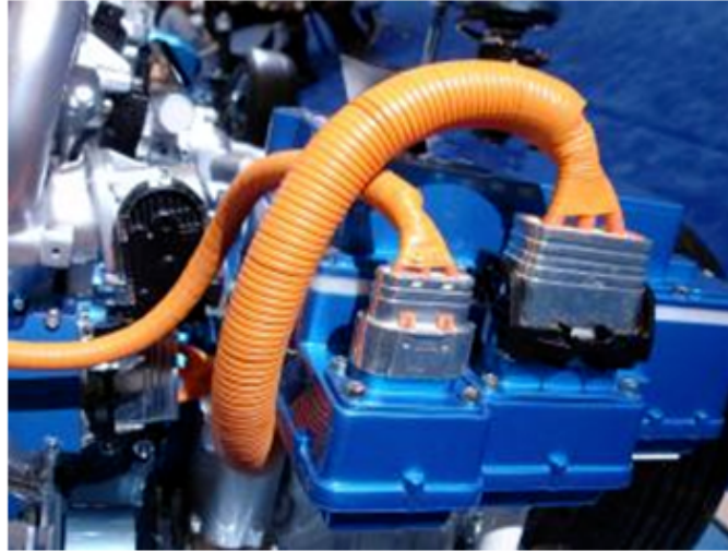
Figure 15: High Voltage wires indicated by orange caps
