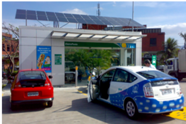
Figure 12: Charging Station run on solar power in Rio de Janeiro, Brazil
