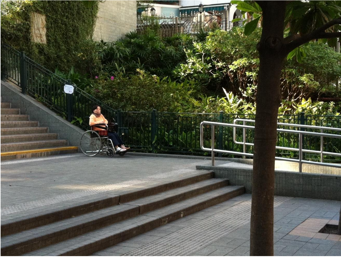
Figure 3: Incomplete handicapped accessibility at Exit A1 of Tsim Sha Tsui MTR Station
