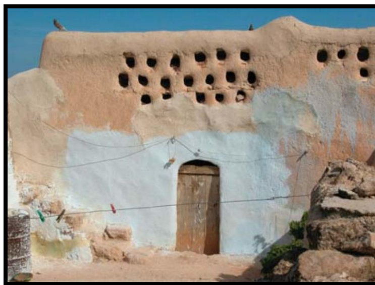
FIGURE 5: MUD WALLS WITH PLASTER RENDERING
