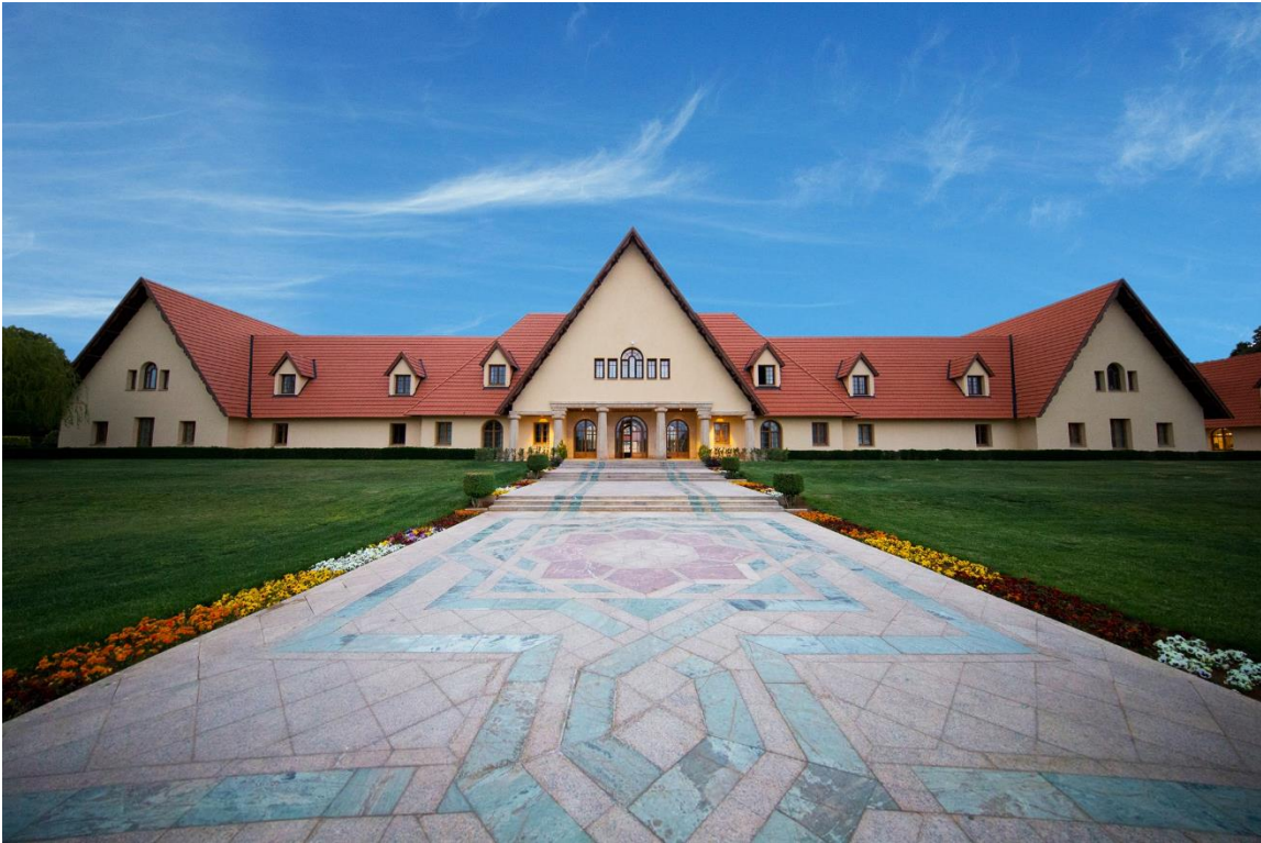
Figure 8: Al Akhawayn University's campus (Al Akhawayn University [AUI], n.d.)
