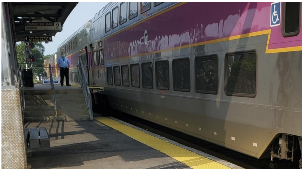
Figure 2.9. Mini High-Level Platform at Framingham Station
