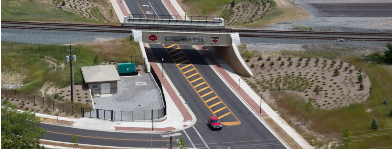
Figure 4.29. Completed Grade Separation in Lima, Ohio (“Railway Engineering Services”, n.d.).
