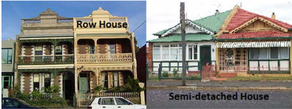
Figure 20 - Semi-detached and Row Houses
