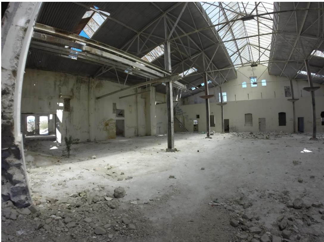
Figure 4.3 - Former Repair Shop Building in Usakos
